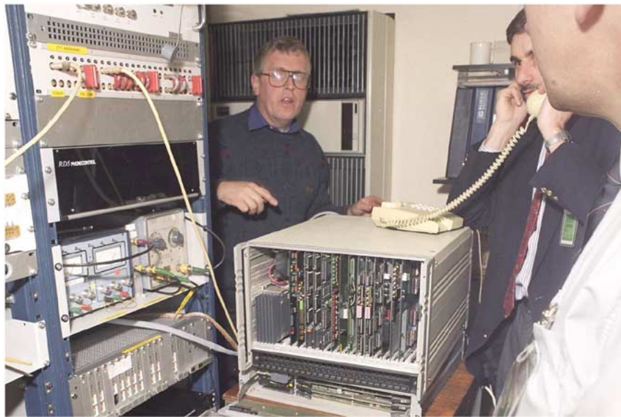
Fig. 6. BBC DVB-T prototype modulator and multiplexer at the Crystal Palace transmitter site in South London in 1996. The system was built for the first DVB-T live transmission. The rack in the center is the BBC DVB-T modulator (from left to right: Nick Tanton, Mark Maddocks, and Chris Clarke).
